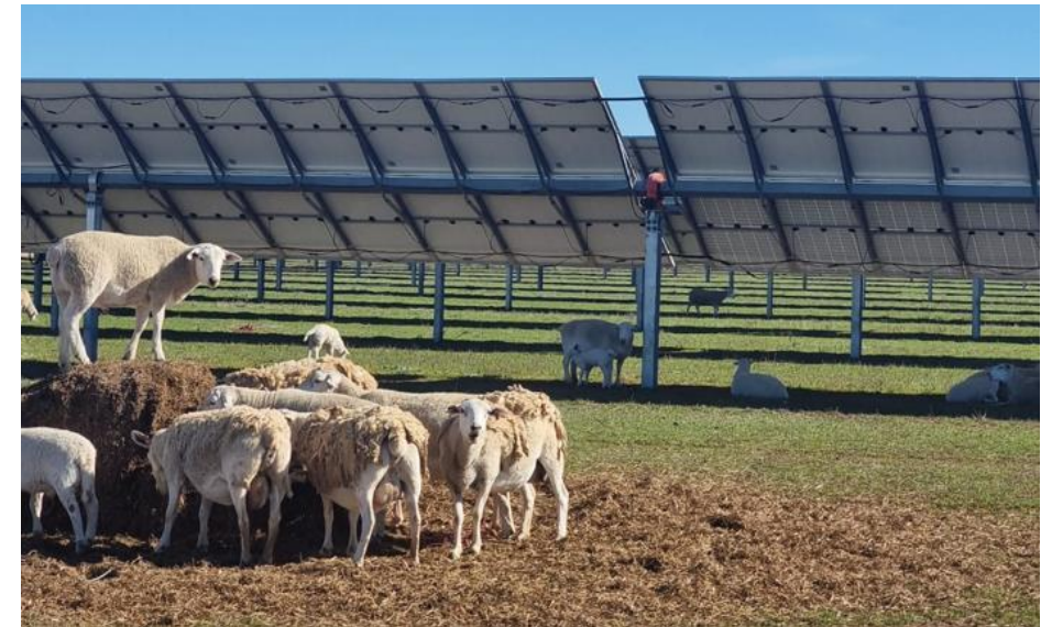
Sheep grazing at a constructed solar farm
