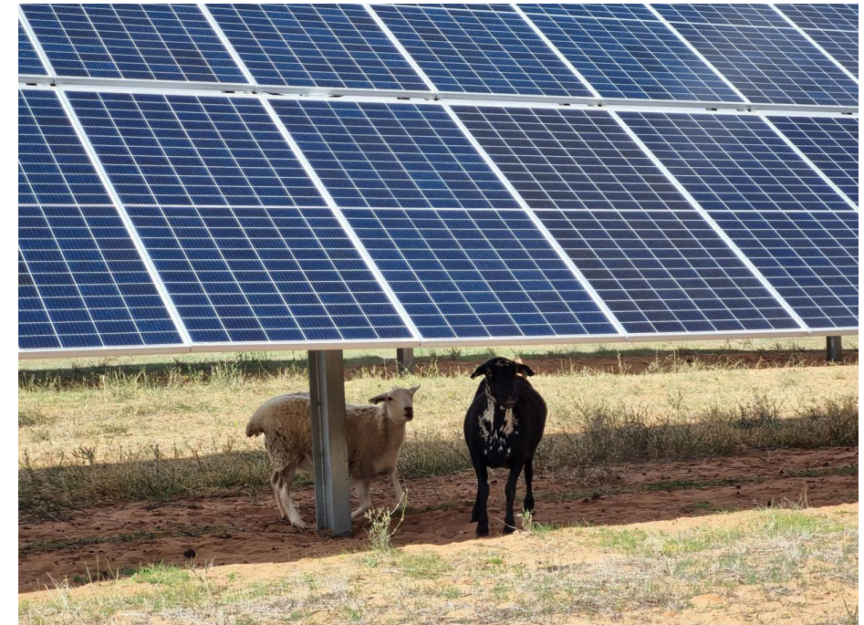
Sheep grazing at a constructed solar farm
