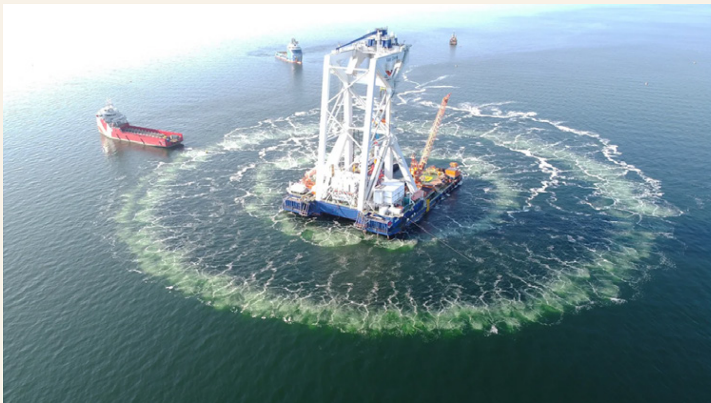
Source: Creating a curtain of bubbles around the area where an offshore wind turbine is being installed can help to minimise the noise - BBC
