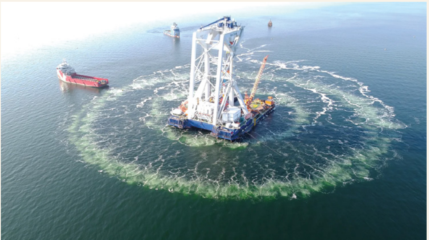
Source: Creating a curtain of bubbles around the area where an offshore wind turbine is being installed can help to minimise the noise - BBC
