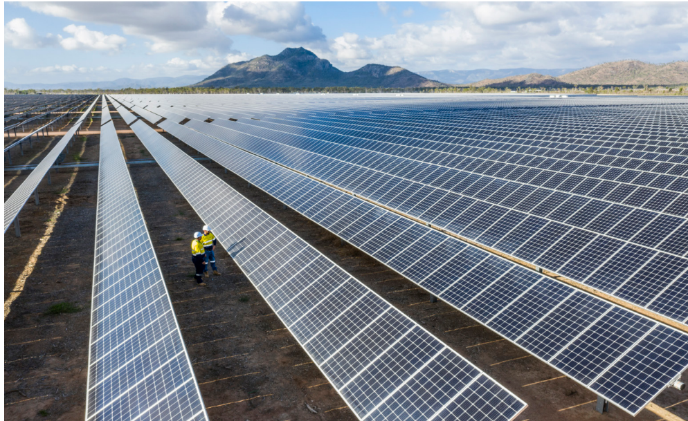
Ross River Solar Farm, QLD
